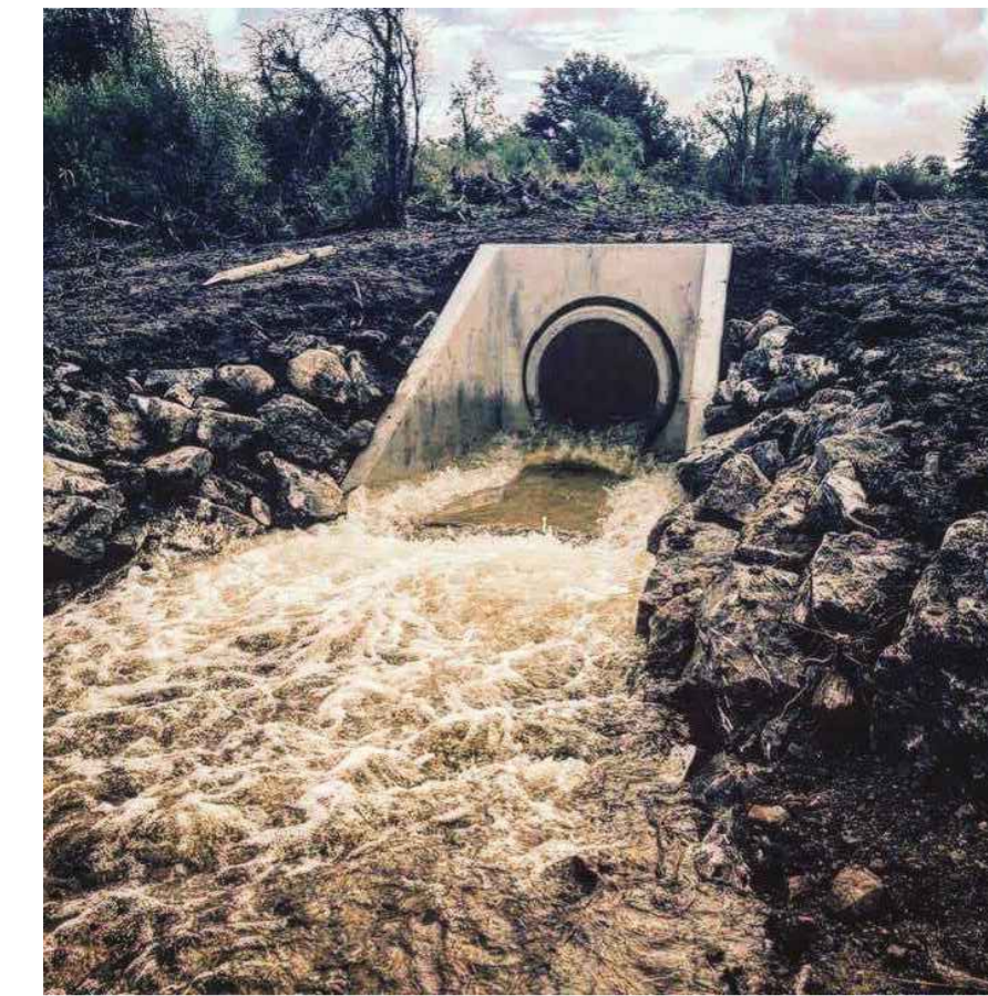
EXAMPLE OF PRECAST CONCRETE PIPE CULVERT
