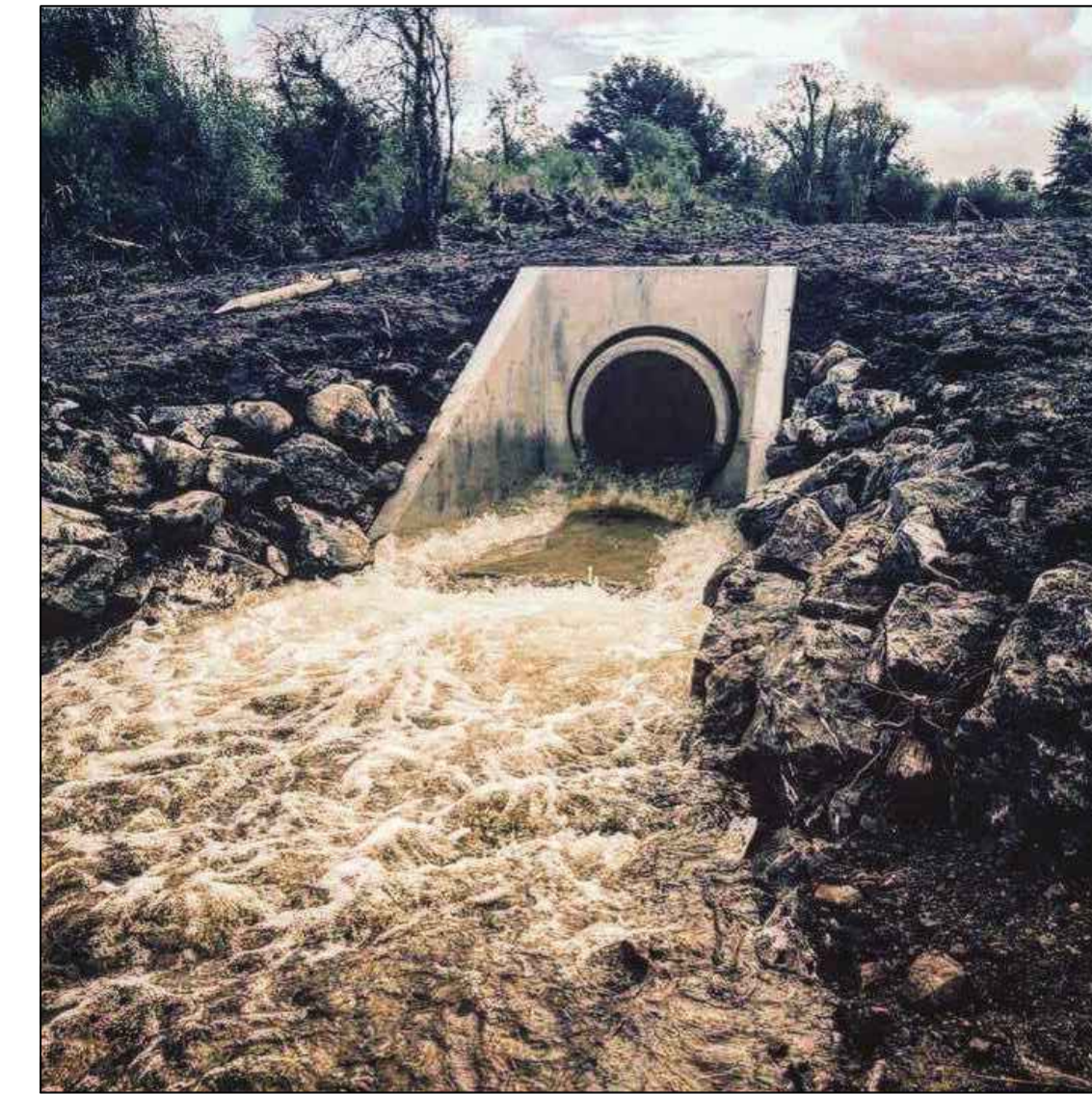
EXAMPLE OF PRECAST CONCRETE PIPE CULVERT
