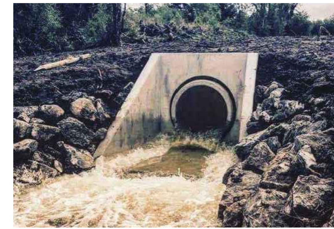
EXAMPLE OF PRECAST CONCRETE PIPE CULVERT
