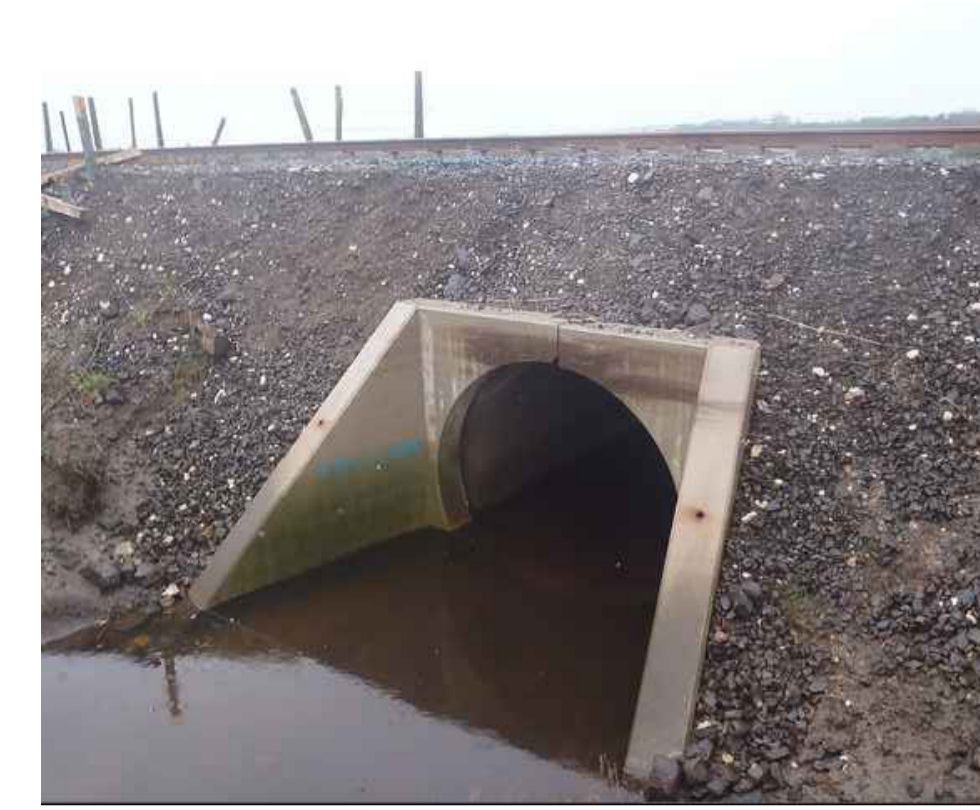
EXAMPLE OF PRECAST CONCRETE PIPE CULVERT
